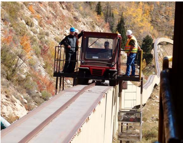
Figure 5. Using Modified All-Terrain Vehicle as Trolley
