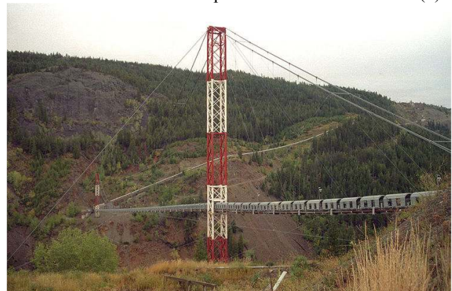
Figure 1. Similkameen Ore Conveyor Bridge in British Columbia, Canada
