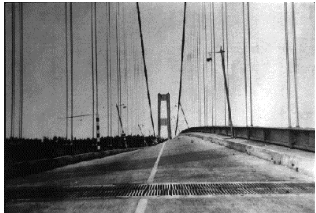
Figure 3. Twisting Motion of Tacoma Narrows Bridge
